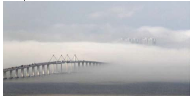
The Picture 4 The Partial Fog is Flowing to the Airport
